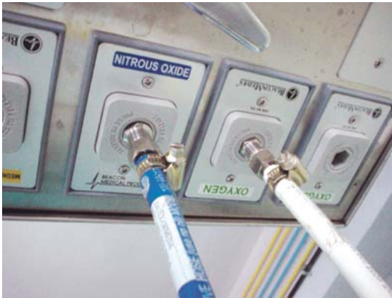
Fig. 4.5: 'Quick coupling' attachments
